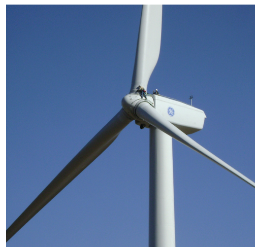
DWP wind generator maintenance crew at work
